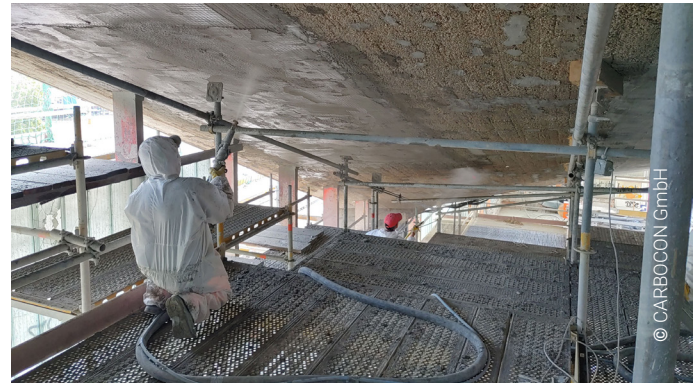
Fig. 2, 3: Restoration project involving the reinforcement of the Hyparschale
