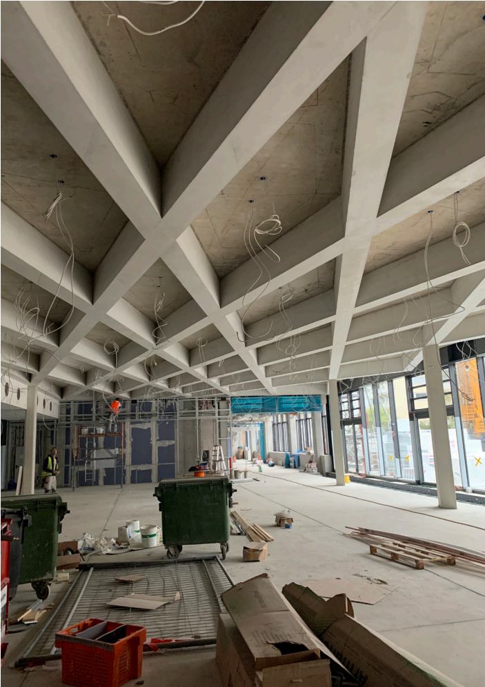
The casino ceiling with lattice work of beams. (©Wulle Lichti Walz)
